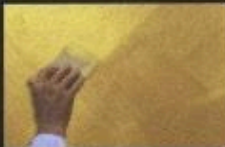
Applicare Heavy Metal con sprayer a pennello associato. Attendere 2-3 ore e ripetere la stessa operazione per la 2 a mano. Apply Heavy Metal coating with sprayer brush. Wait 2-3 hours and repeat the same operation for the 2nd coat.
