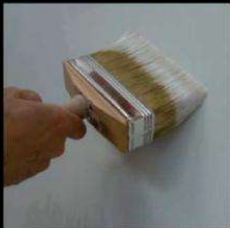
1- Cover Primer applicazione a pennello (1 mano) Application of Cover Primer with brush (1 coat)
